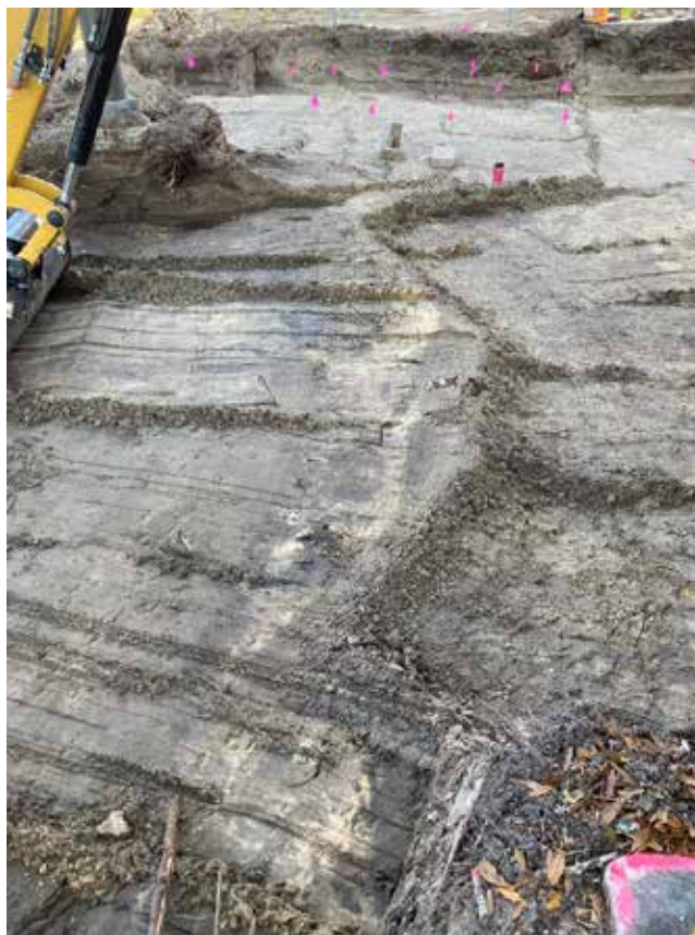
Figure 59 View of utility trench-sewer during mechanical stripping, looking east.
